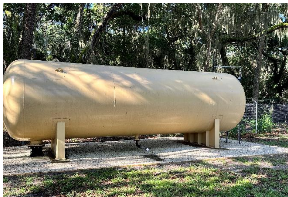
Hydropneumatic Tank 1
